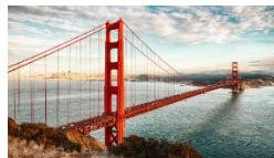
Golden Gate Bridge
