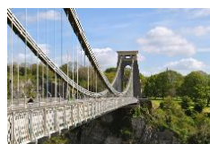
Clifton Suspension Bridge
